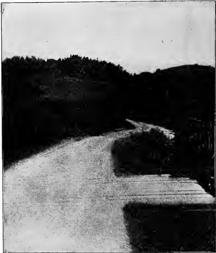
FIG. 292. — Horizontal shifting of a road in California. Before the 1906 earthquake this road was straight. (Sinclair.)
